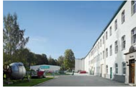
Thalheim presspaper plant
