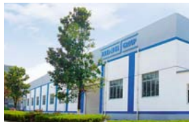
Zhangjiagang solar plant / China
